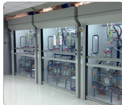
An installation of six 30 litre jacketed reaction systems in Shanghai, China
